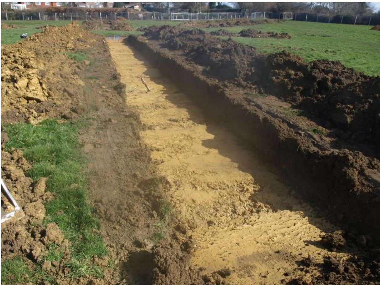
Plate 4: Looking north east at trench 17
