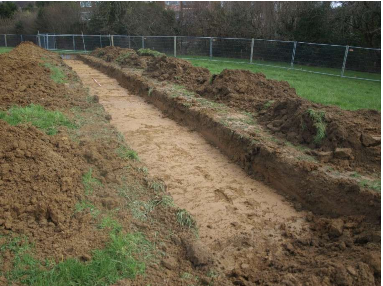
Plate 10: Looking east at trench 45
