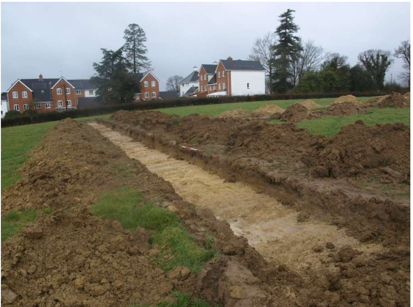
Plate 2: Looking north west at trench 6
