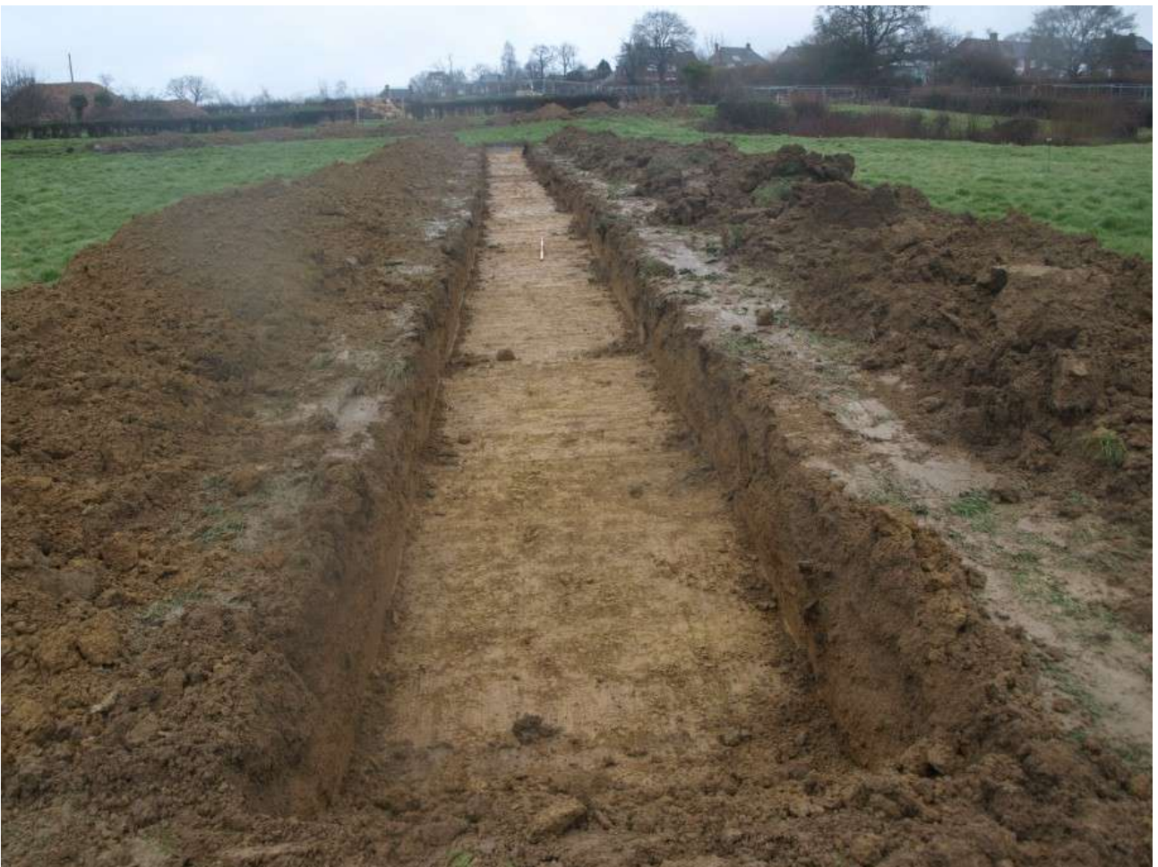
Plate 8: Looking north west at trench 34
